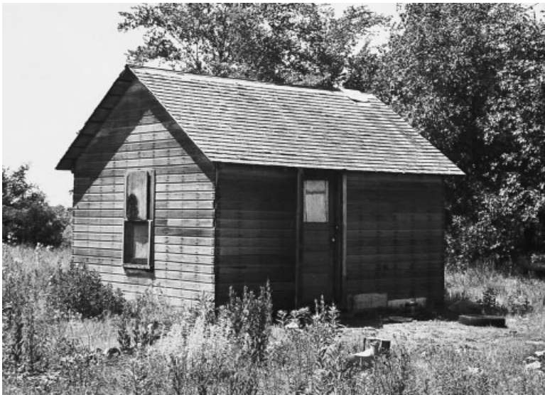
Figure 6.2 A typical 12'-x-14' house built for the Prairie Island Dakota in the 1930s (photographed in July, 1960. Minnesota Historical Society Photograph Collection)
