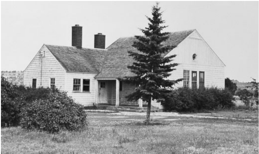
Figure 7.1 The Prairie Island Community Hall in 1960 (Minnesota Historical Society Photograph Collection)
